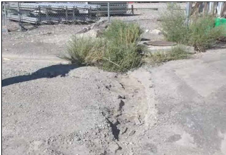
Manhole where lid intermittently blows off.
