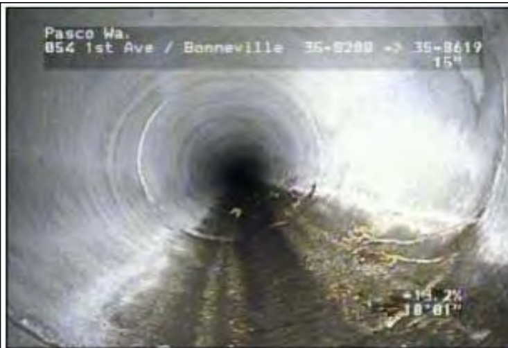
Example of root penetrations.
