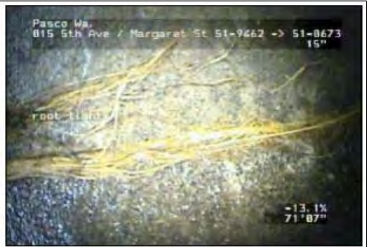
Roots in pipe tributary to Sylvester North to be relined.
