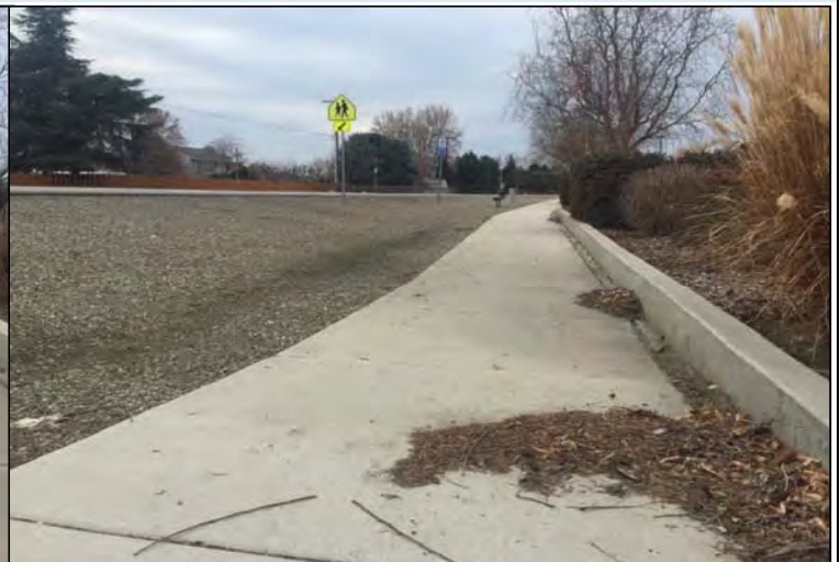
Accumulated debris due to runoff.
