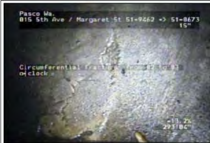
Fracture in pipe tributary to Sylvester North to be relined.
