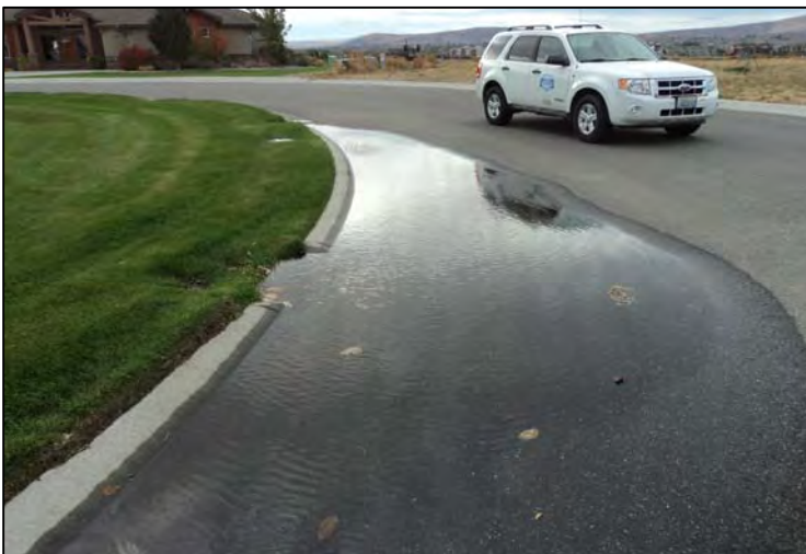
Ponding at inlet to existing infiltration swale.
