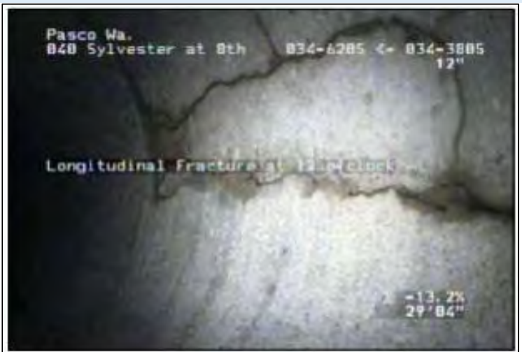
Fracture in pipe tributary to Sylvester South to be relined.
