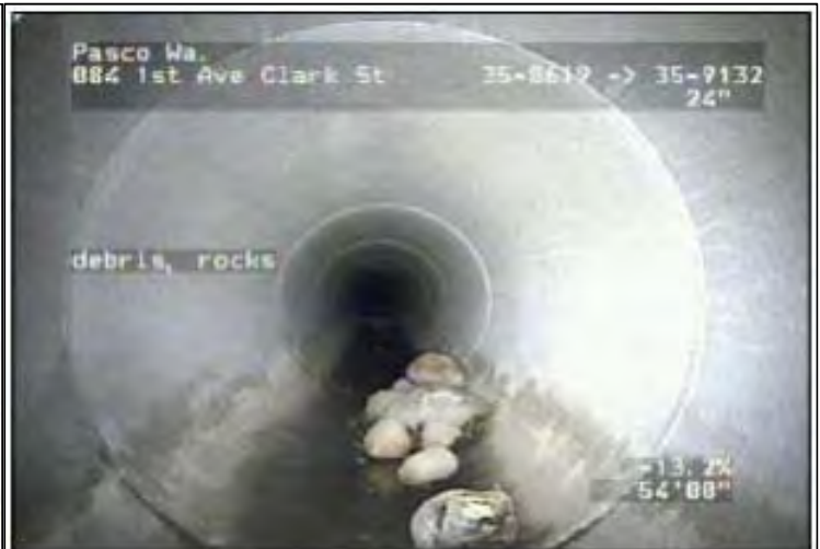
Example of accumulated rock debris.
