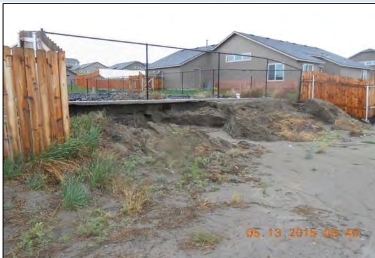
Embankment damage on the east side of the pond.
