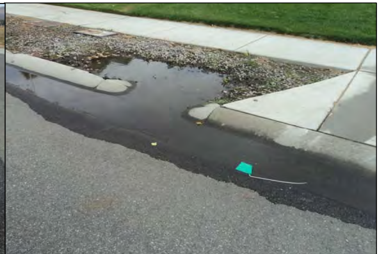
Ponding at curb cut to infiltration area.
