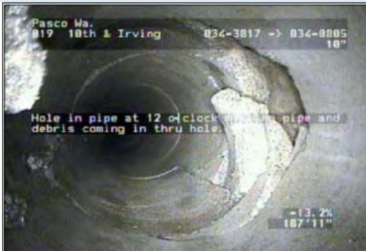
Condition of pipe tributary to Sylvester South to be replaced.
