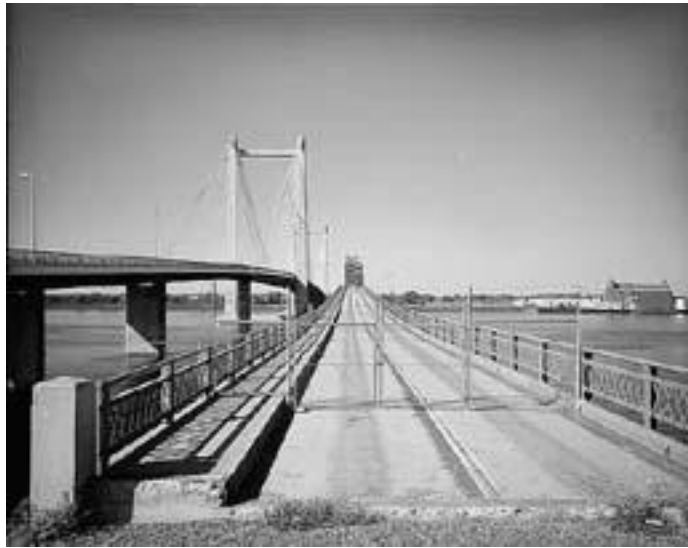
Pasco-Kennewick Columbia River Bridge/Benton-Franklin Inter County Bridge (now demolished) shown in 1980 next to the newly-constructed Ed Hendler cable-stayed bridge. (photo courtesy Historic American Engineering Record)
