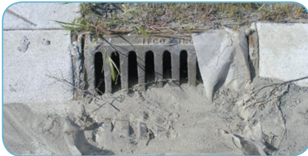
Sand in gutter and catch basin in a construction area.
