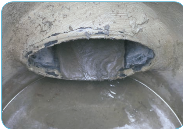
Sand inside ex-filtration trench pipe inside catch basin.
