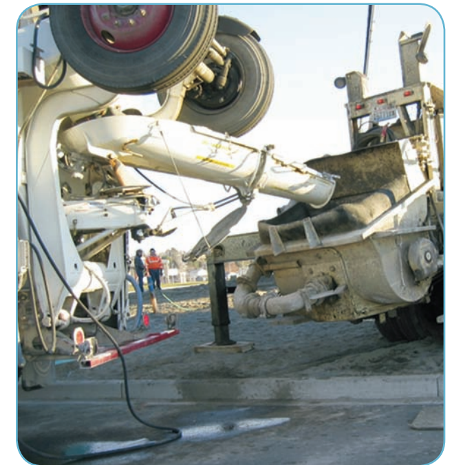
Potential for concrete to spill into gutter.
