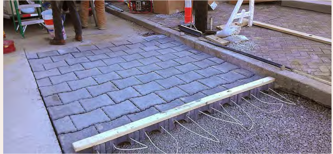
PERMEABLE PAVEMENT HELPS STORMWATER TO INFILTRATE ON-SITE
